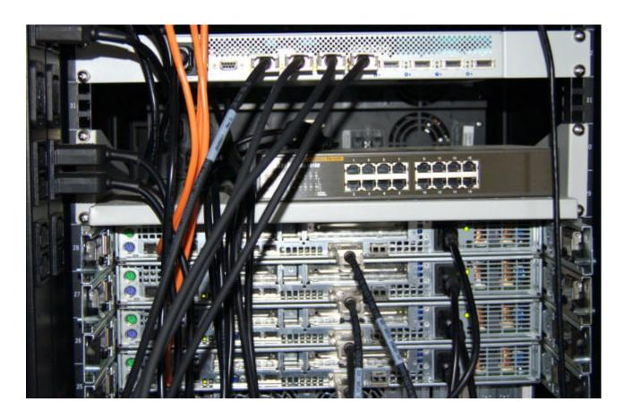
The upper unit is the Infiniband switch
